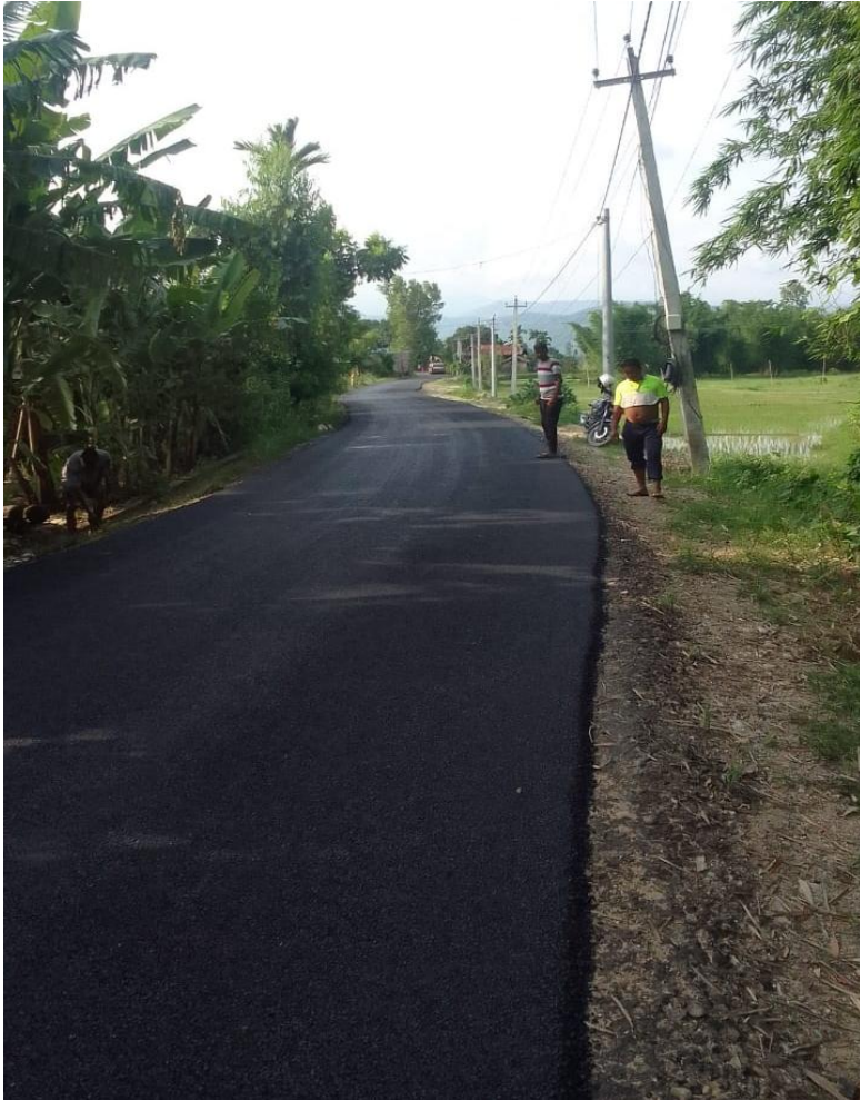
Upgrading of Ward No. 9, B.P. Chowk, Sukrabare, 10 No. Ward Office, West Bakainiya to Debdhar
