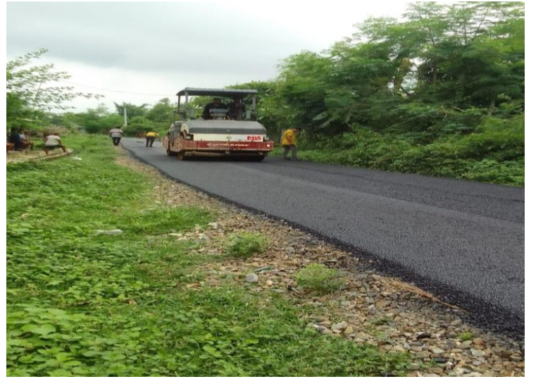
Upgrading of Ward No. 9, B.P. Chowk, Sukrabare, 10 No. Ward Office, West Bakainiya to Debdhar 9& 10
